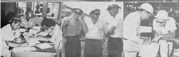
SOME OF the 320 men and their supervisors involved in the project are shown as they begin their day's duties, preparing to put on coveralls, poring over diagrams and figures in the mobile office, and discussing progress of the twelve-day project.
